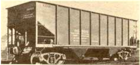
Loads of hopper cars are dropped from bottom.
