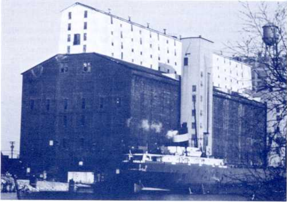
The Great Northern Elevator, built in 1897 by James J. Hill, is now called the Mutual Elevator and is an adjunct to the Pillsbury Flour Mill. It is of a unique design having steel bins enclosed in a brick sheath.
