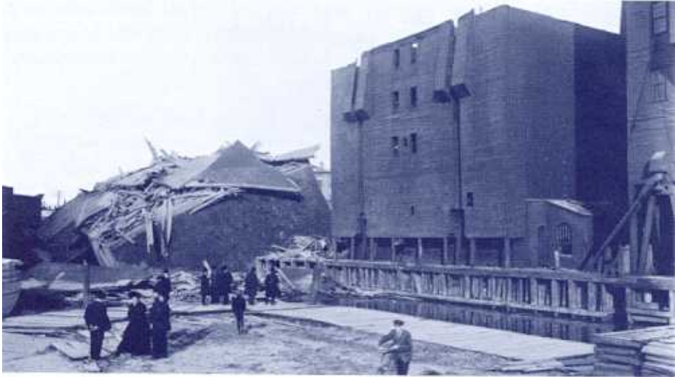
The Ontario Elevator on the Evans Ship Canal after it collapsed in 1904.
