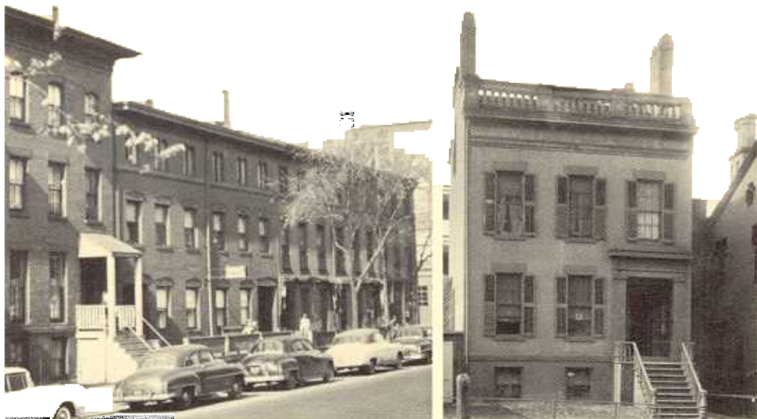
Left: Row houses on Swan and Michigan Streets c. 1855. Right: Many free-standing houses had wooden or cast iron balustrades at the edge of the roof. The first floor is a half-story above the grade.
