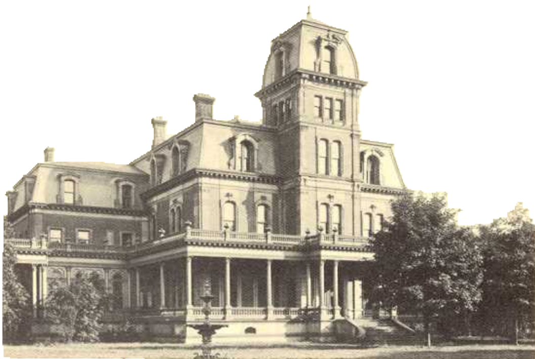
The William G. Fargo home had an expansive mansard roof and open porches.
